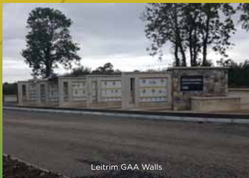
Entrance View of Walls
